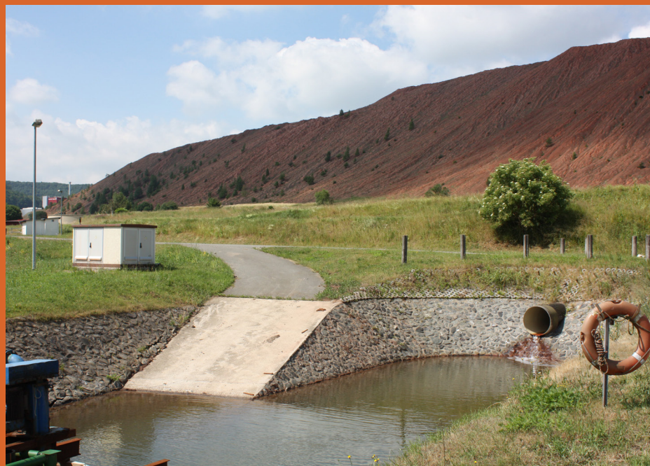
→ Image: Uncovered potash waste dump with drainage water collecting system in Germany
