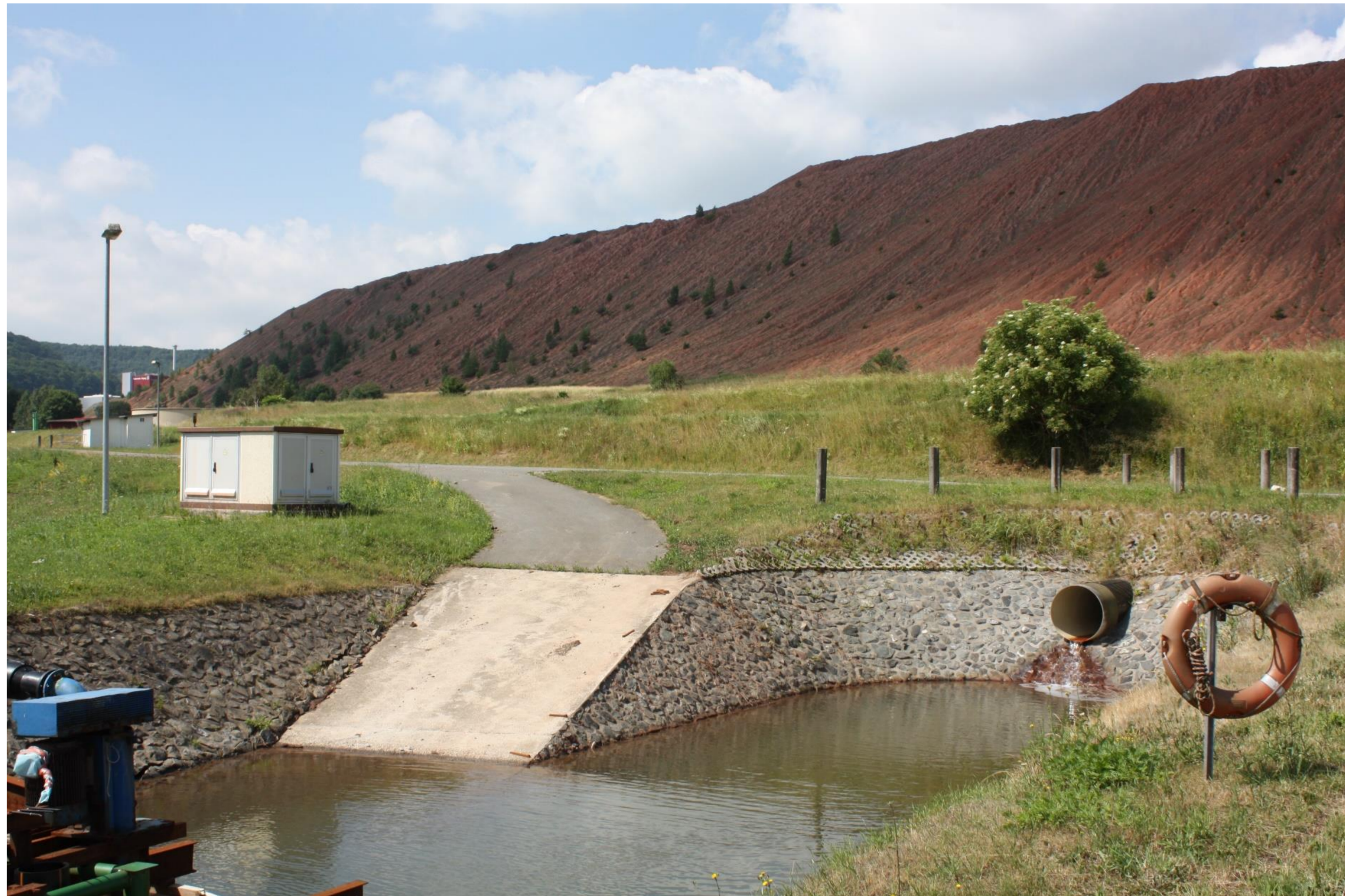
Fig. 1: Uncovered potash waste dump with drainage water collecting system in Germany
